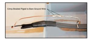
**12.** Carefully push connected wires into Junction Box and secure cover. Ensure a drip loop in the exiting cable under Junction Box to prevent seepage.
