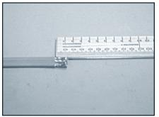
**End Termination Step 13:** Cut back overjacket 0.5" (12 mm).
