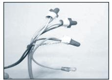
**Step 10:** The incoming power cable should also be provided with a drip-loop before it enters the enclosure. Connect the power conductors to the cable leads. Connect the incoming supply ground wire to the cable braid and to the green ground wire. Crimp the ring terminal to the other end of the green ground wire and then connect it to the grounding screw on the lock-ring.
