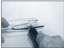
**Step 5:** Skive outer matrix material from conductors with a utility knife.
