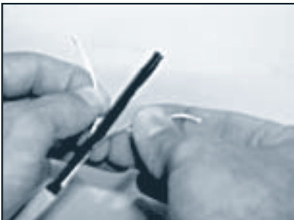
Step 5: Peel exposed wires back from center matrix and cut center matrix away, leaving bare conductors.
