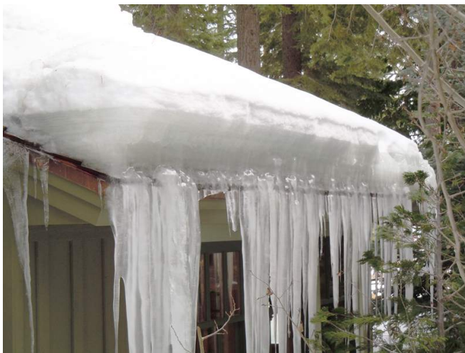
24" thick ice dams are not uncommon at Tahoe
