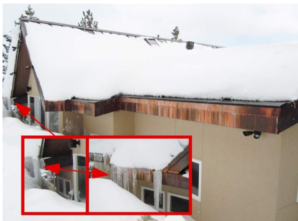
PRO to Right. Inset Shows Adjacent Unheated Roof Up Close
